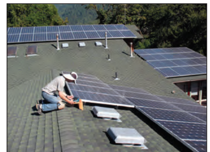
Top: Project Manager Jim Zoellick checks the shading profile for the Weitchpec solar electric array. Bottom: Research Engineer Kyle Palmer tests the interactive touch screen display in the lobby of the Weitchpec Tribal Office. Photo credits SERC.
