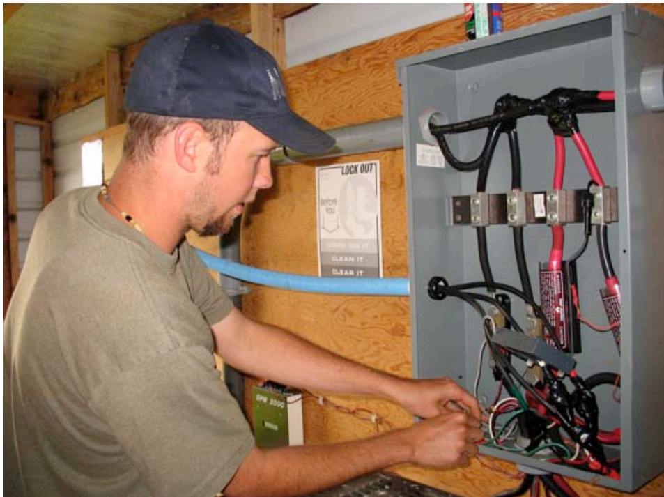
Figure 10 UNPEPP intern Matt Smith installs a HOBO data logger to measure residence power use.
