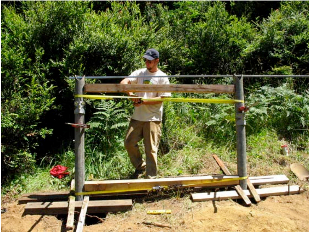
Figure 3: UNPEPP intern Matt Smith spacing the rack poles before pouring concrete.
