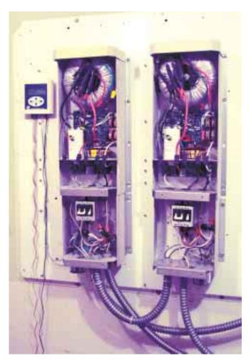
Advanced Energy's AM100 Inverter Monitor (left) and the interior of the GC-1000 inverters.
